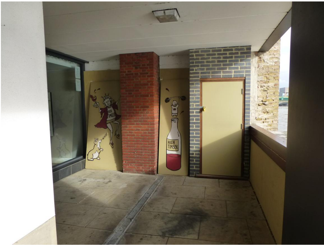
Entrance to East-west section of covered walkway at Sir John Lyon House
