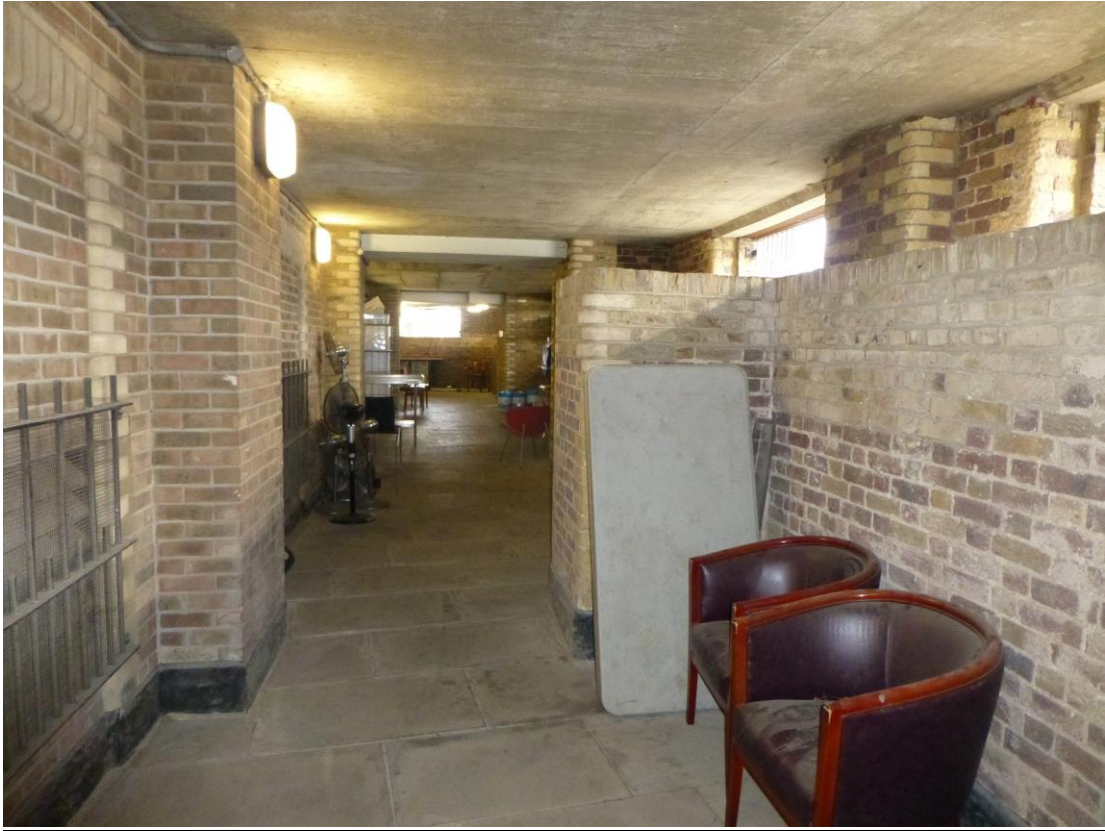
East-west section of covered walkway
